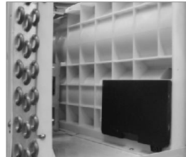
Figure B – Vent Filter Removal
